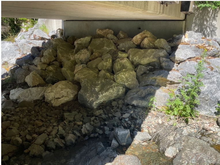
Right Bank Abutment when facing downstream
