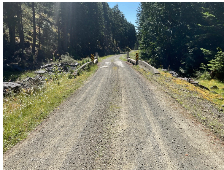
Approach from Right Bank when facing downstream
