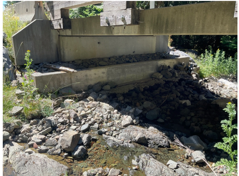
Left Bank Abutment when facing downstream
