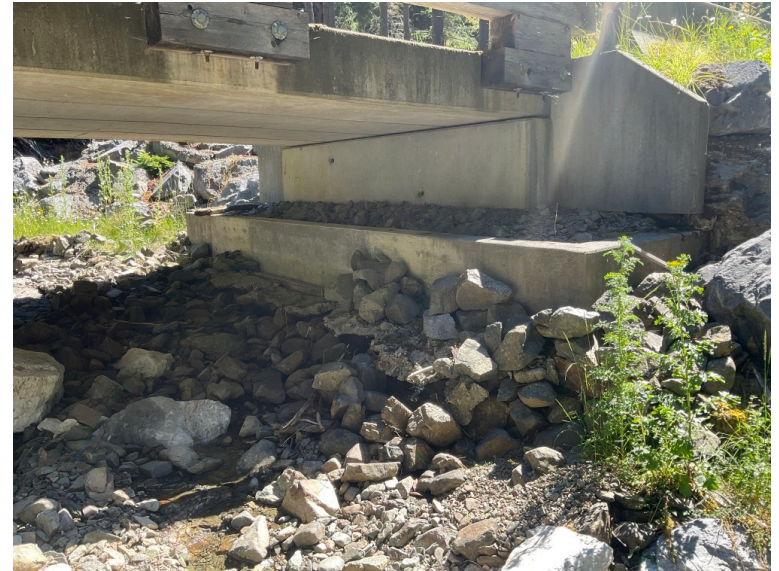
Left Bank Abutment when facing downstream
